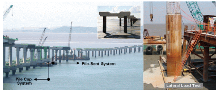
Figure 5. Lateral load test on piles with pile-bent system
