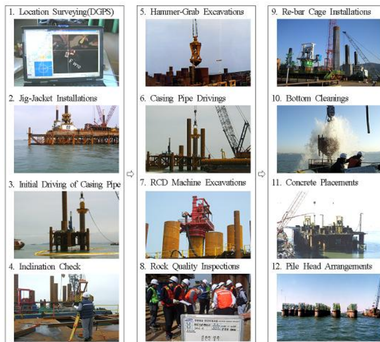
Figure 4. Construction steps for piles
