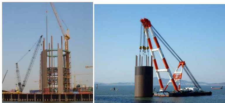
Figure 13. Fabrication and transportation of the dolphin cell
