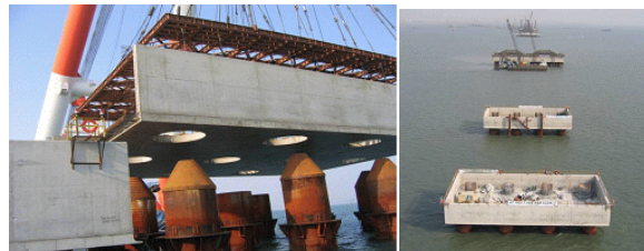
Figure 6. Installation of pile cap using PC House method
