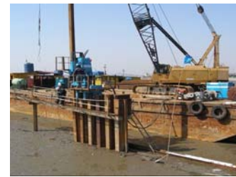
Figure 22. Push-in type sheet pile installation machines
